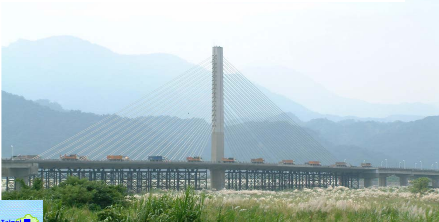
Gi-Lu Cable-Stayed Bridge, Chi-chi, Taiwan Span: 120m (L) + 120m (R)
