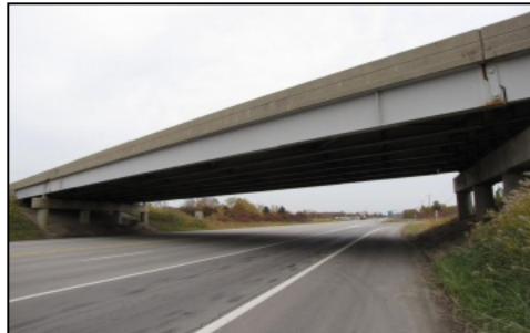
Fig. 2 Testbed bridges: Telegraph road bridge (Monroe, Michigan)
