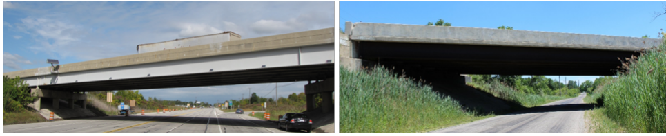
Figure 2. Telegraph Road Bridge (left) and Newburg Road Bridge (right).
