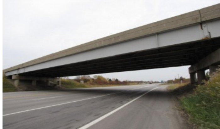
Figure 2.12 Telegraph Road Bridge (Monroe, Michigan)
