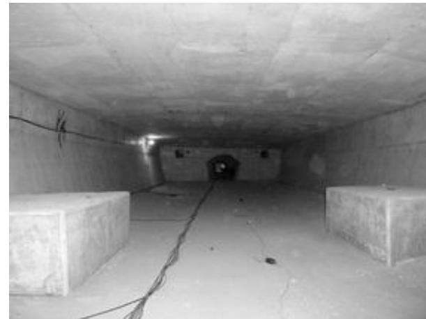
(c) Interior of the box girder
