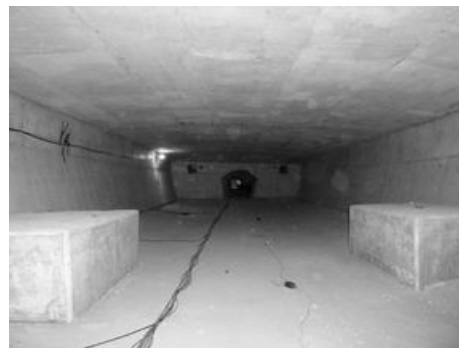
(c) Interior of the box girder
