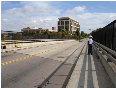
(b) View of the bridge deck
