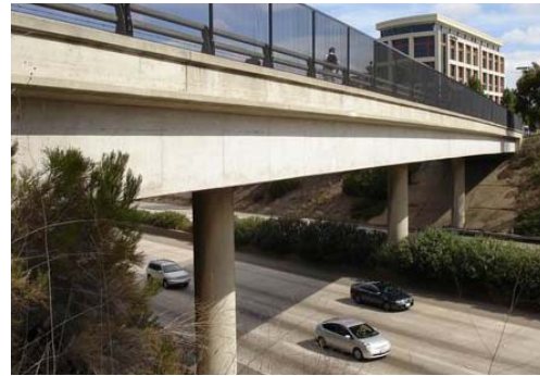
(c) Side view of the bridge over Interstate 5
