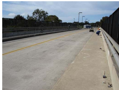
(c) One side of bridge deck with wireless accelerometers mounted
